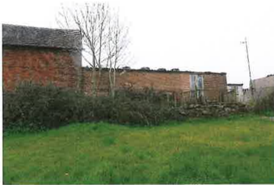
Flat roof section
