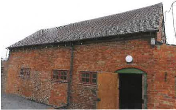
Front of building
